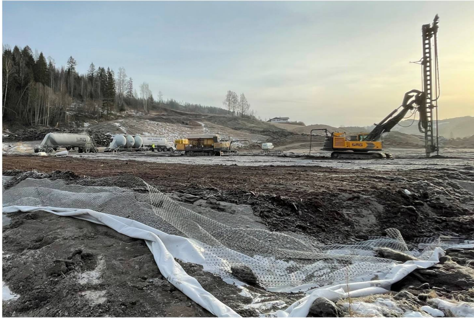
Figure 7 Soilmixing performed by SMG. Credit T. Bjørhusdal.
