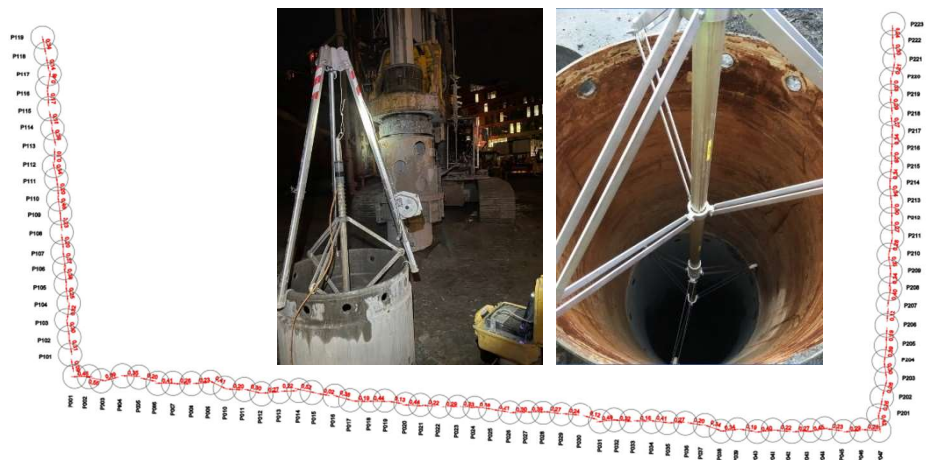
Figure 11 Result of deviation measurements at hole bottom, showing 100 % overlap.
