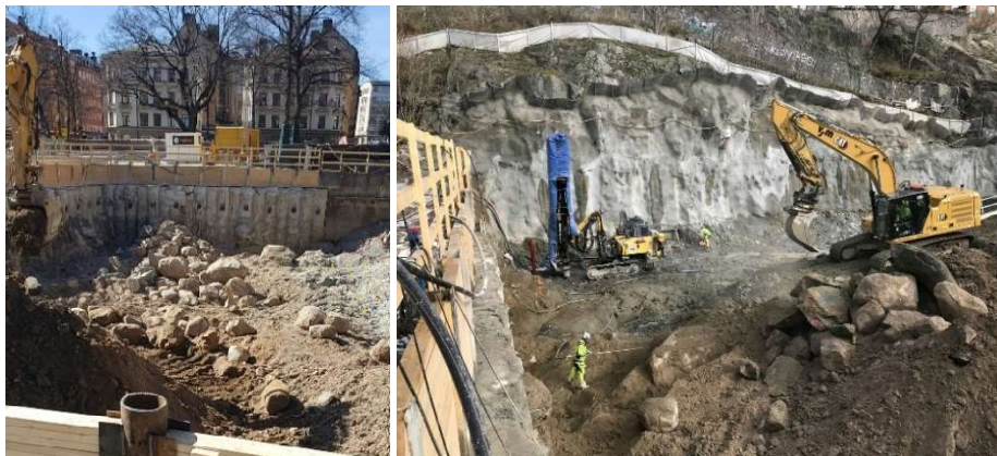
Figure 7 Pictures showing the extent of boulders and of large boulders (>630 mm).
