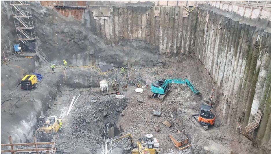
Figure 15 Secant pile wall, facing east and south.
