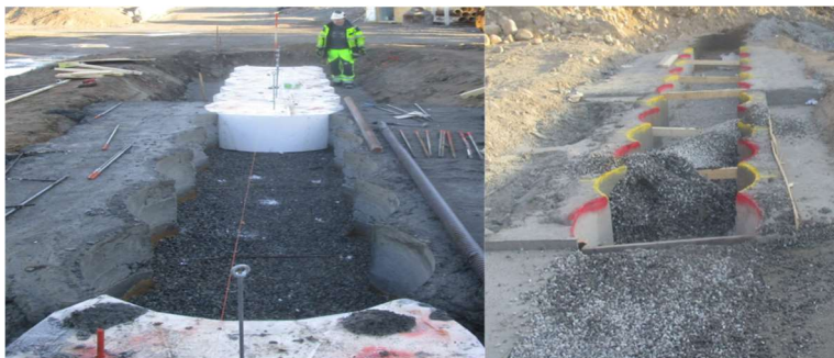
Figure 10 Pictures showing a typical drilling template for aiding alignment.
