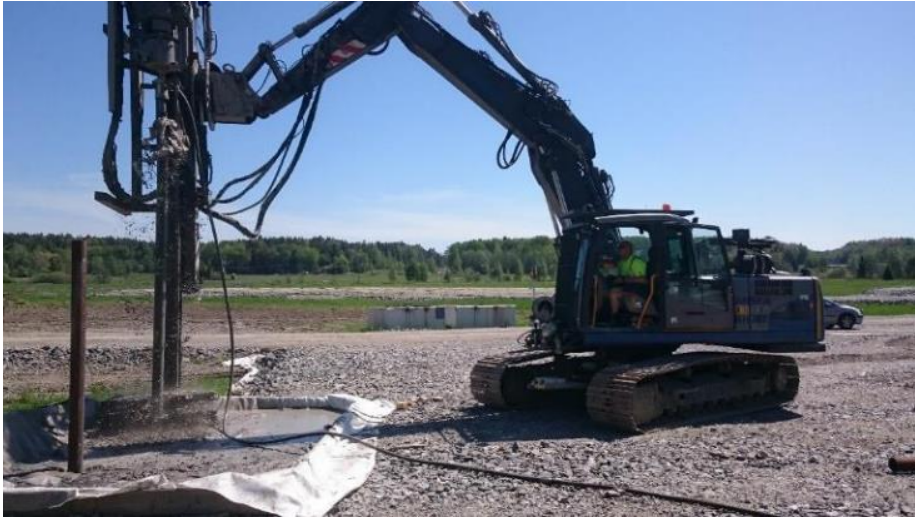
Figure 2. Drilling of a steel pile with an air driven DTH hammer.
