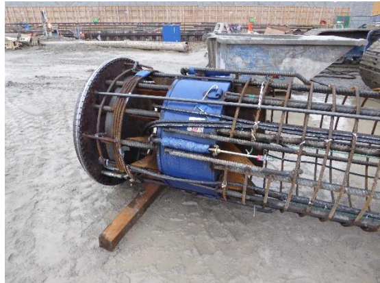
Figure 2: Flat-jack and O-cell mounted on reinforcement cage.
