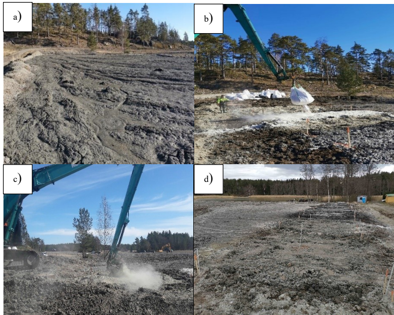
Figure 1. Field test: a) dredged spoil before stabilization, b) adding binders, c) mixing, and d) test field ready.
